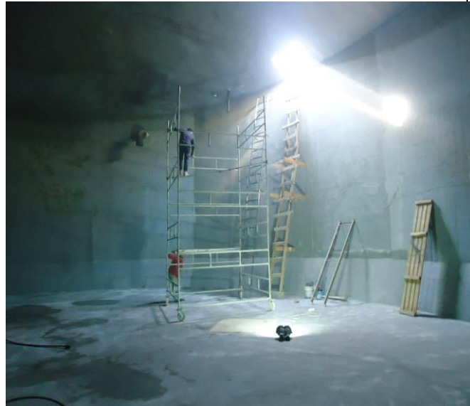
Internal insulation works
