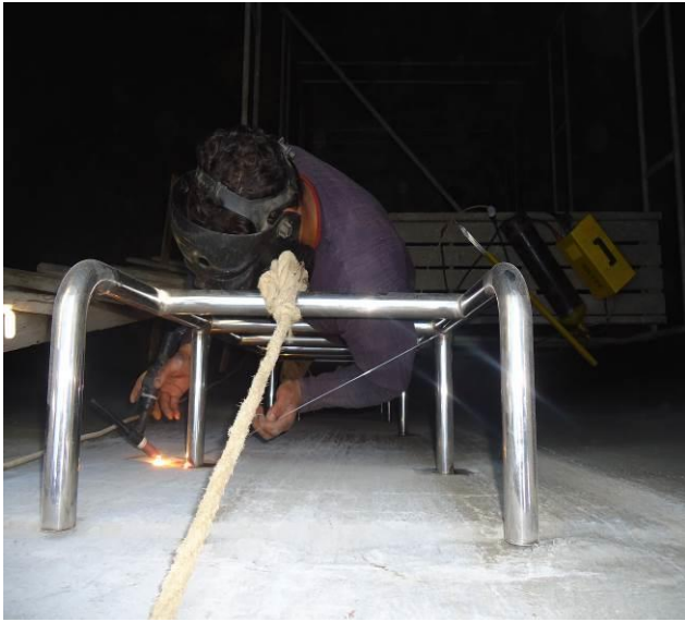
Internal stainless steel ladder works
